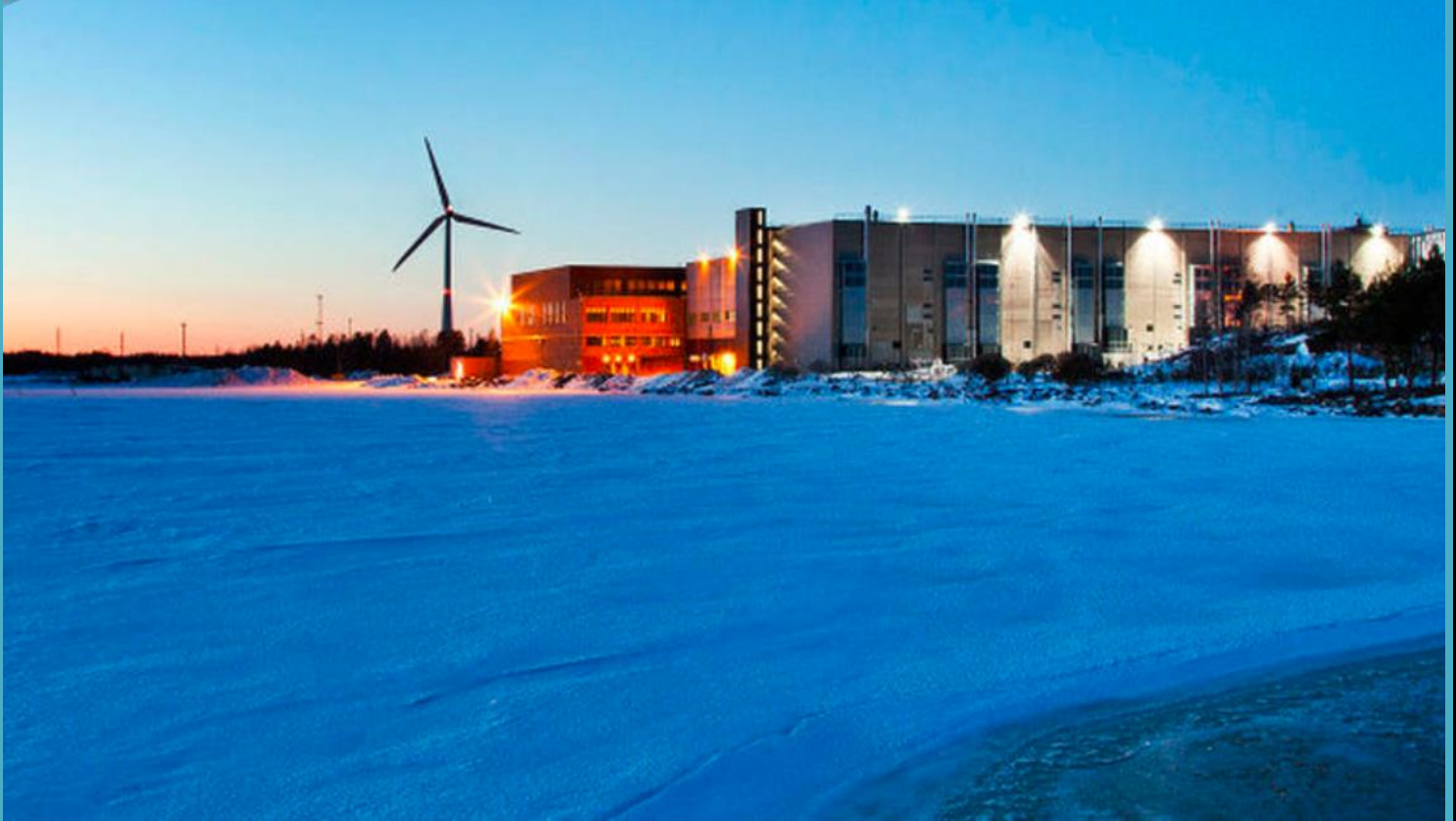
Figure 3. Google's Hamina Data Centre with PUE of 1.1
